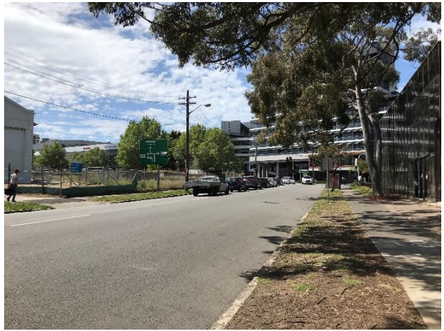
View to the east along McEvoy, fronting the 840 Bourke Street building and Dank Street South to the left
