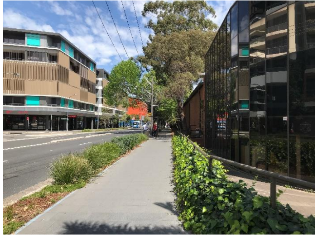
Looking South along Bourke Street within the frontage of the site
